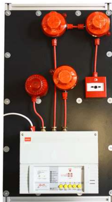
Conventional 4-Wire System 1 used on the fire alarm system installation training course
