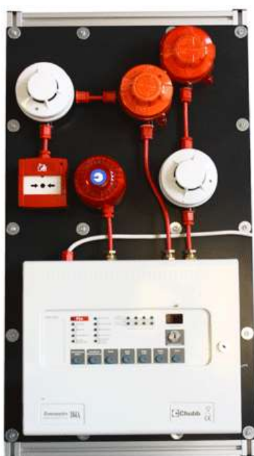
Analogue addressable System 1 used on the fire alarm system installation training course
