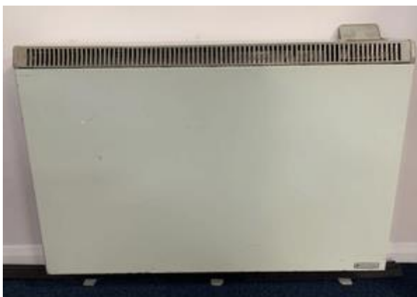
One of our storage heaters. We perform the necessary isolation, inspection and testing of this too.
